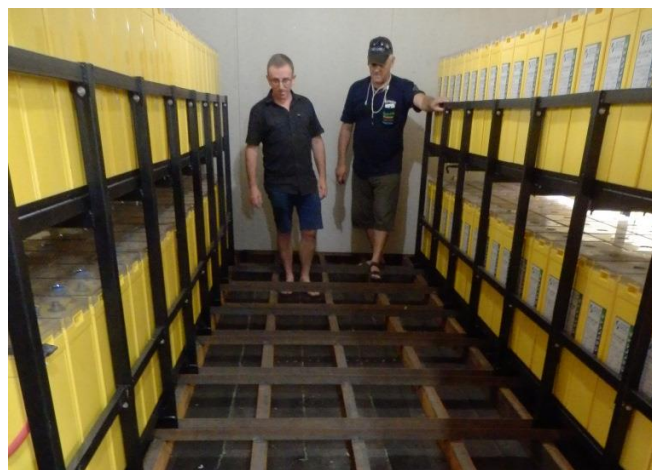
Raised reinforced battery bank
